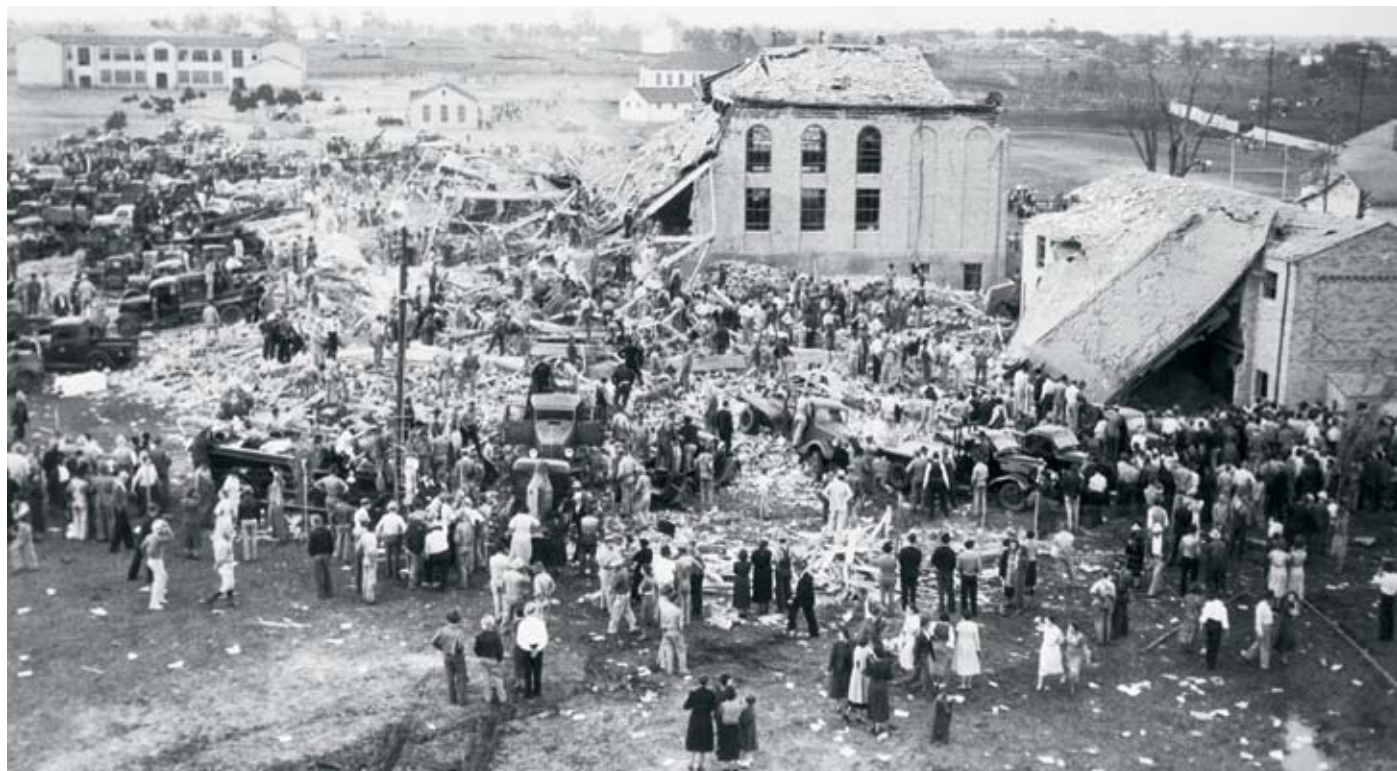
IN 1937, AN EXPLOSION AT A SCHOOL IN NEW LONDON, TEXAS, WAS ATTRIBUTED TO A GAS LEAK CAUSED BY FAULTY ENGINEERING. APPROXIMATELY 300 PEOPLE DIED.
