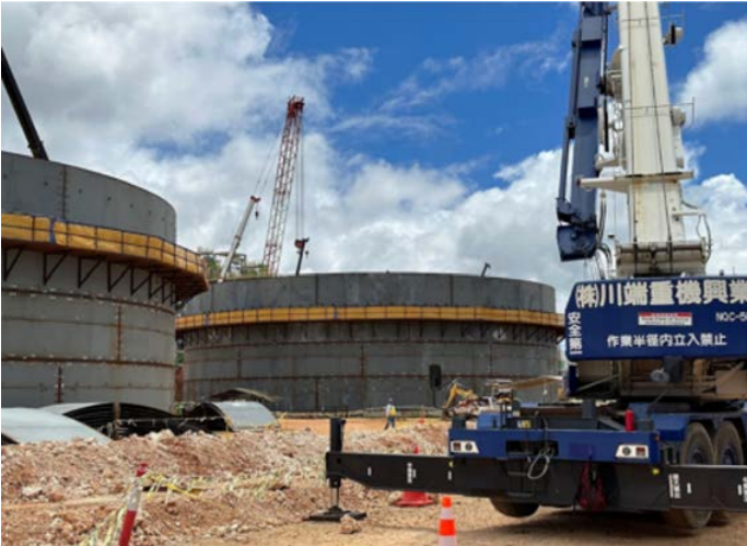
ULSD Tanks A&B, May 8, 2023
